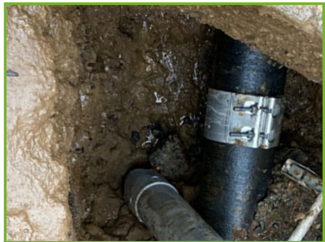
Repair band installed
