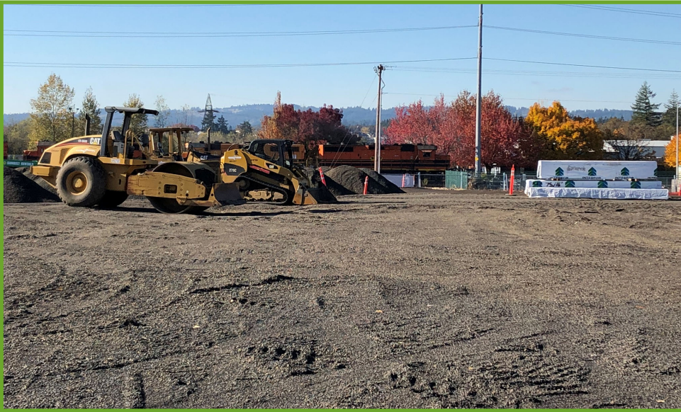
Site has been graded and rock placed over the work areas.
