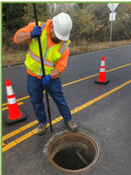
Chipping out the manhole
