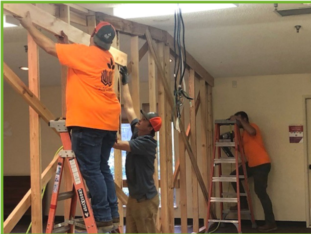
Shoring up at the Kiva building
