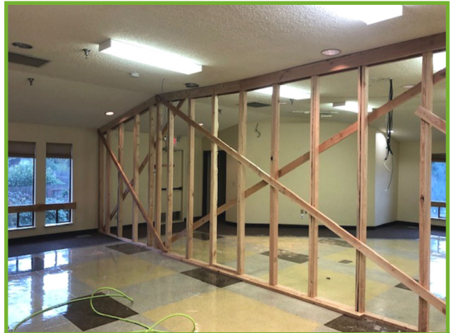
Finished support at the Kiva
