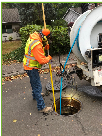
Tim jetting the sewer line
