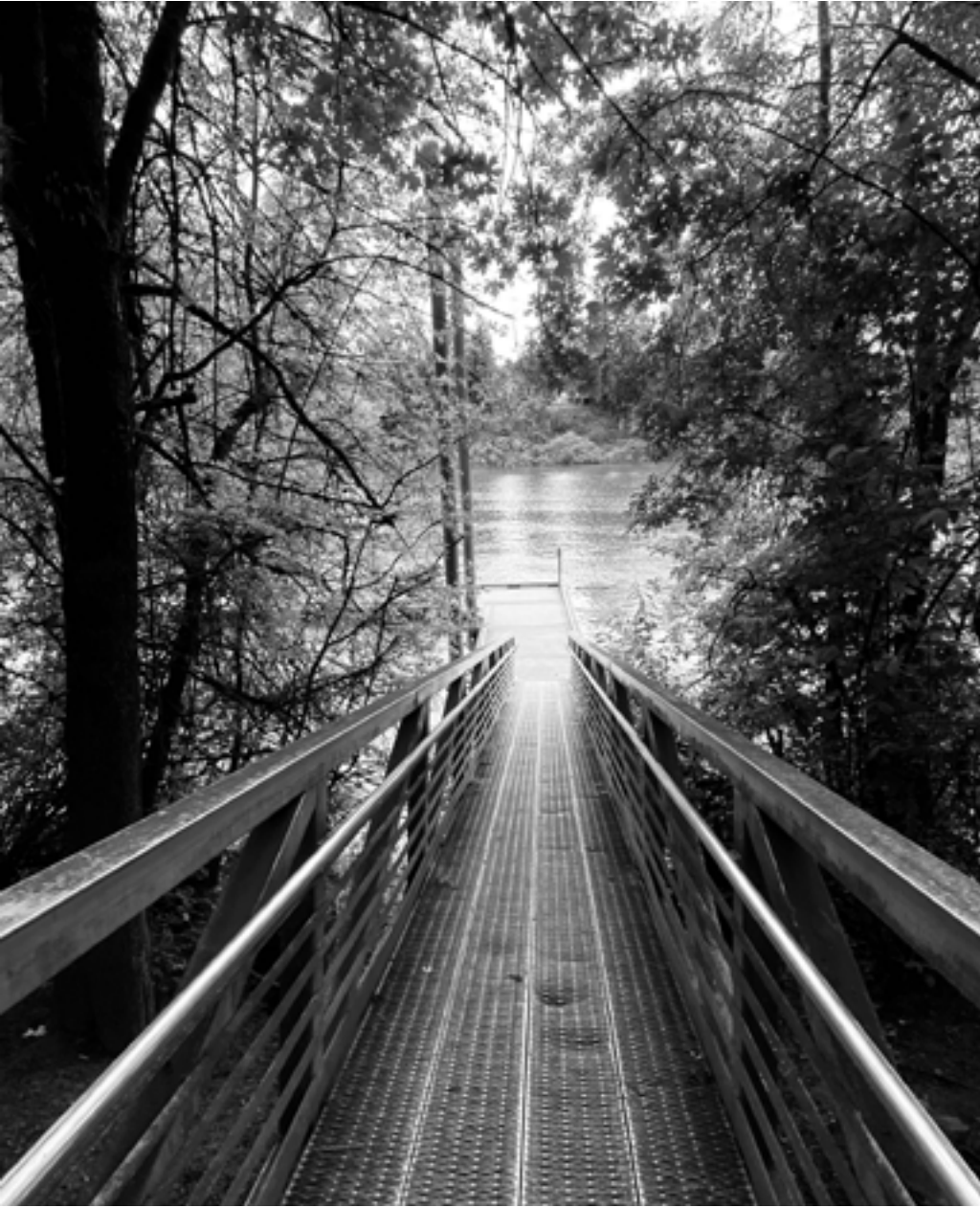
Metal walkway leading to boat dock on Willamette River at Memorial Park in Wilsonville. Credit: Eddie Gao
