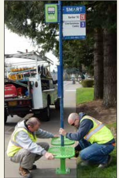
Public Works staff installs bench.
