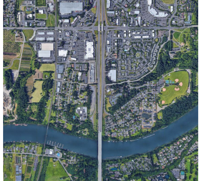
Fig. 1 Aerial of Wilsonville and the Willamette River
