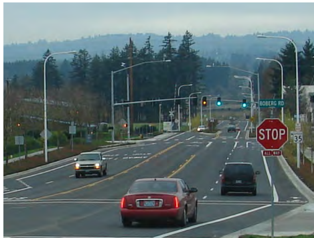
Example of a Major Arterial - Boeckman Road looking west towards Boberg Road and 95th Avenue
