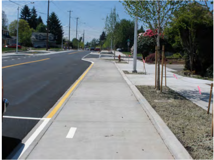
One-Way Cycle Track on Cully Boulevard in Northeast Portland. Cycle tracks are typically protected from motor vehicle traffic by parked cars, raised curbs, or other physical buffers.
