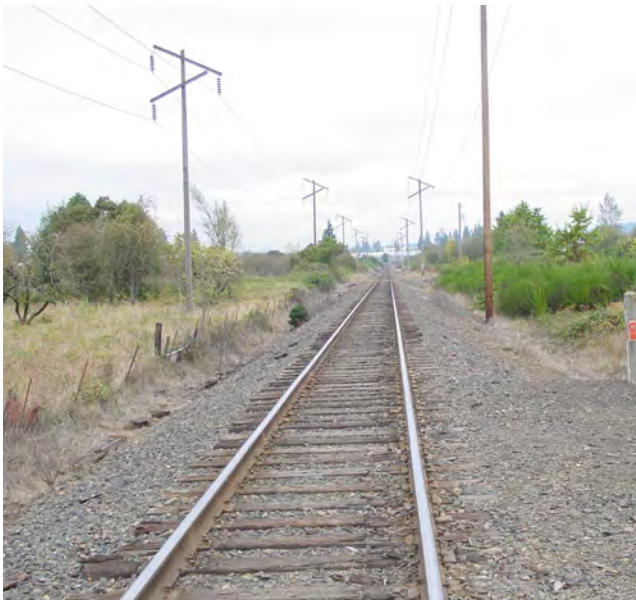
Portland and Western's Oregon Electric rail line runs north/south through Wilsonville and serves as an important freight and commuter rail corridor. However, it also creates a barrier to travel for other modes due to limited crossing locations.
