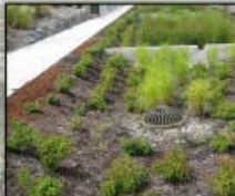
1. STORMWATER MANAGEMENT FACILITY
