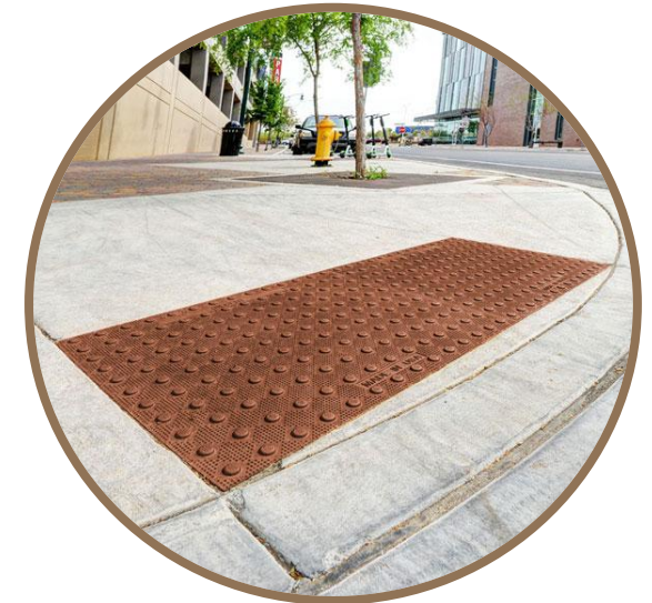
Neenah Foundry Quick Connect cast iron tactile pad for Signature locations
