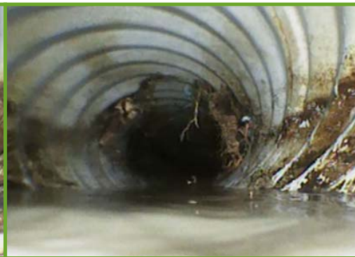
After— line cleared
