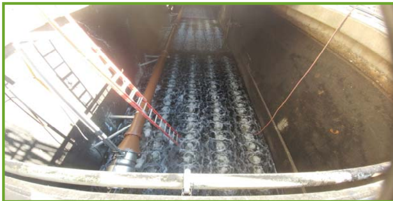
Testing new air diffusers which add oxygen to the activated sludge
