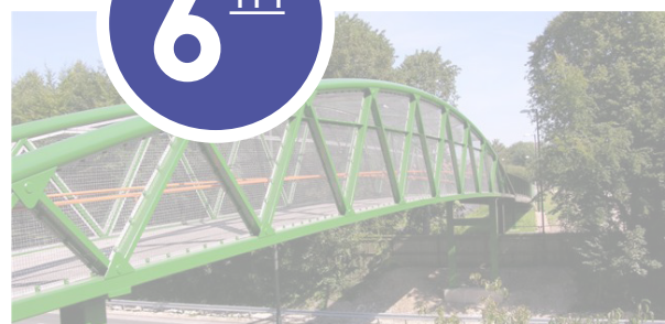
COLOR OF BRIDGE SUPPORT
