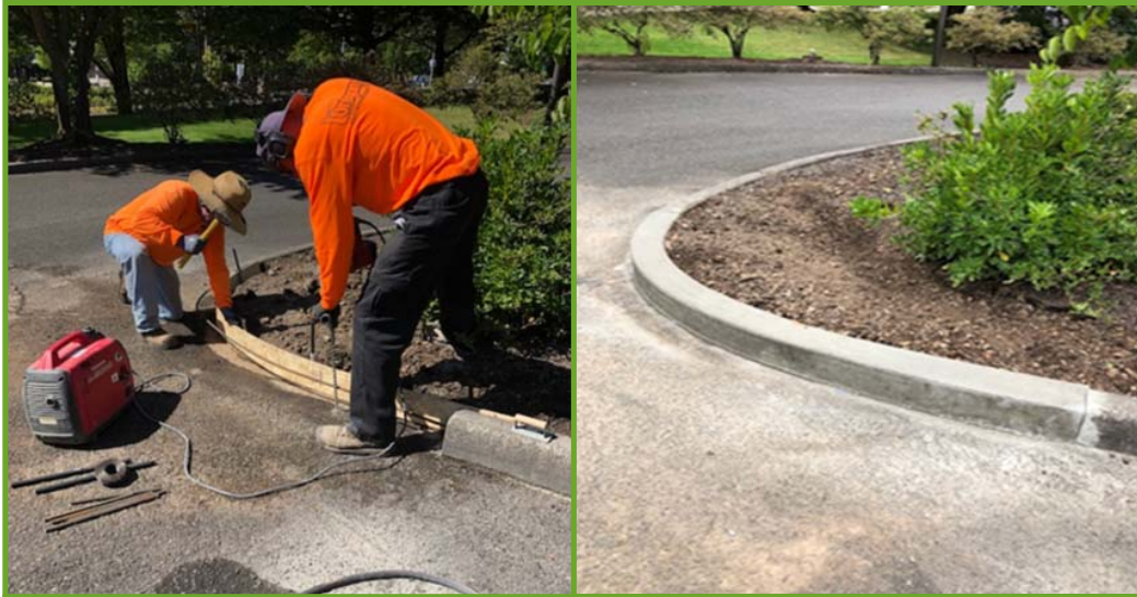
Daniel Morena and Mike Pierce tackle curb repair
