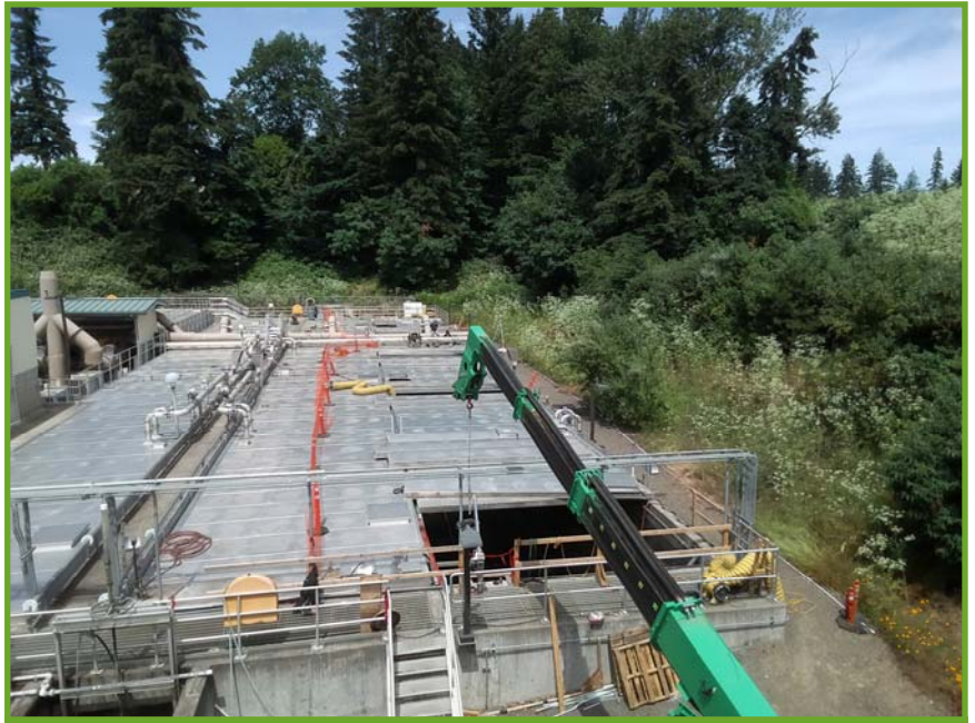
Crane removing cover panels over aeration basins
