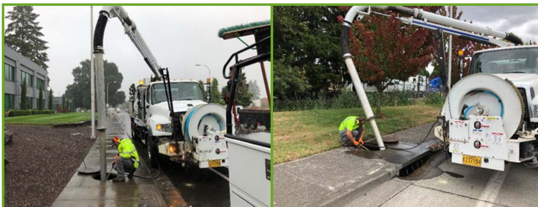
Performing scheduled catch basin cleaning
