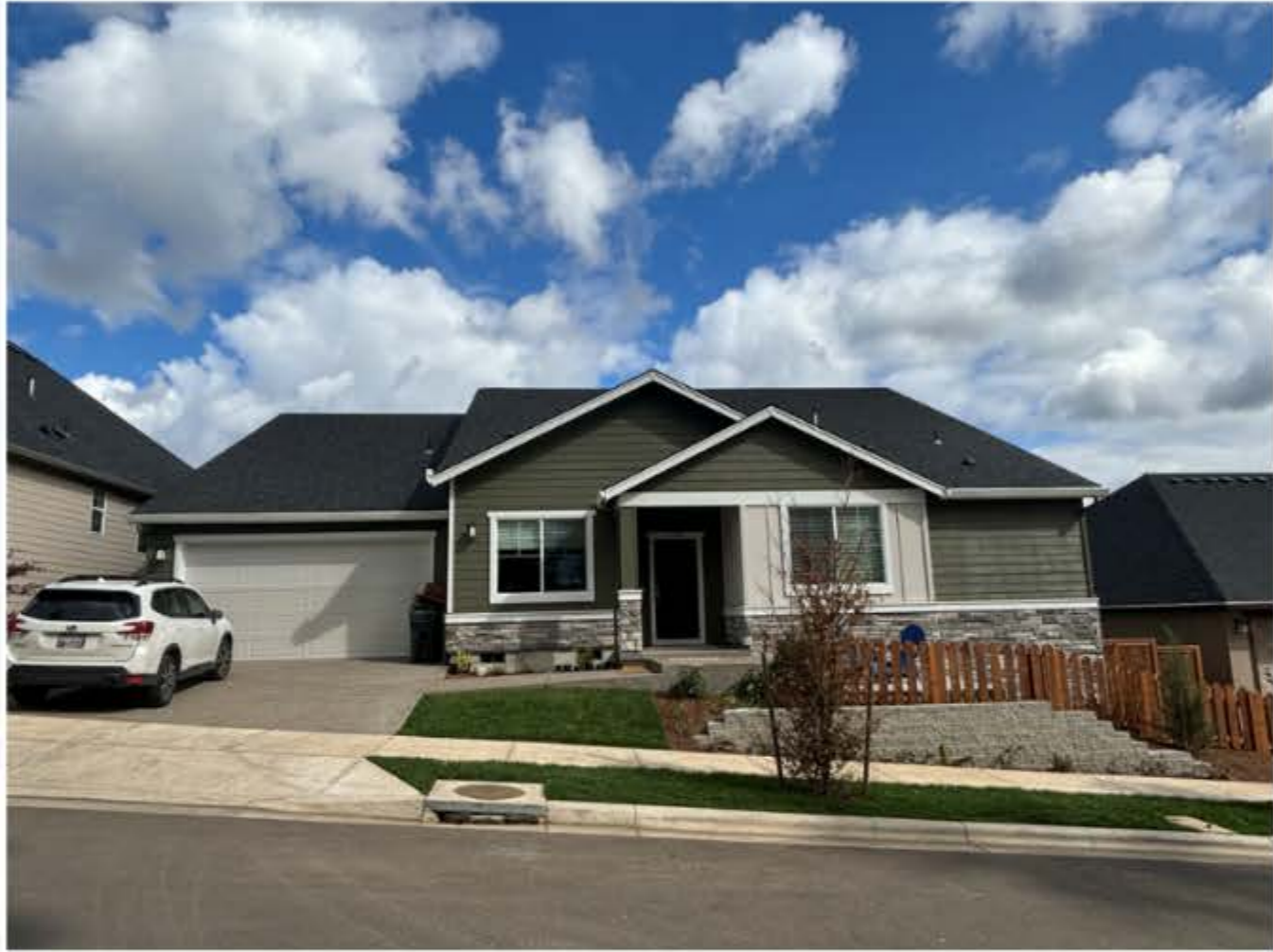
Figure 9. Single level home in Clermont (Villebois).
