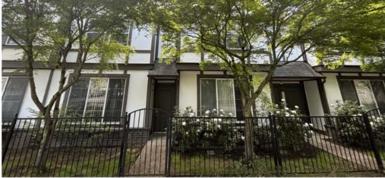
Figure 7. Ground floor apartments in Arbor Villebois (Renaissance Court).
