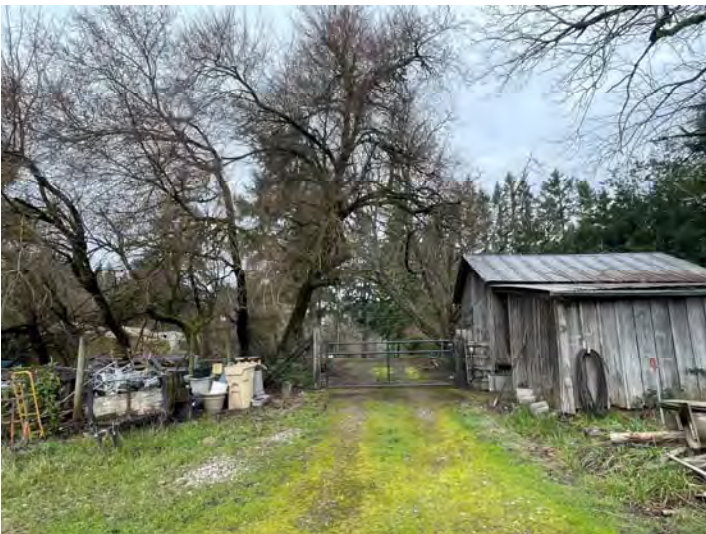
Photo C. View of some of the storage buildings associated with the home facing the northwestern corner of the study area.
